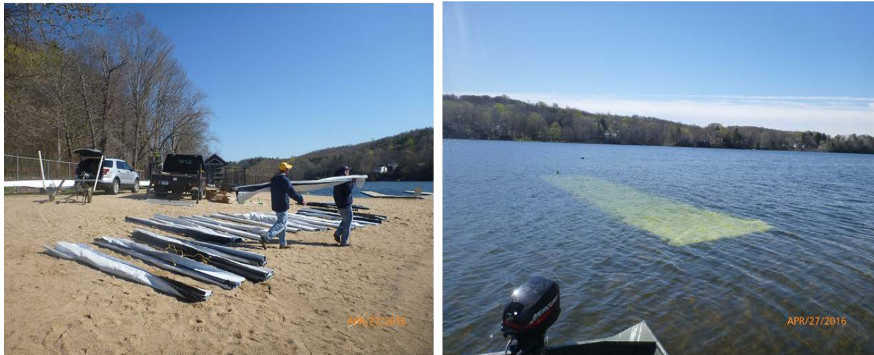
Figure 18. Benthic barrier being installed in Lake Quonnipaug, Guilford, Connecticut.
