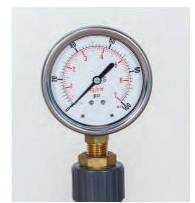
Air testing of PEX piping must follow the manufacturer's instructions.
