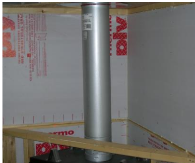
Manufactured fireplace installed with air barrier (gypsum board, Thermoply, or equivalent) in place. All seams caulked, taped, or sealed with expansive foam.
