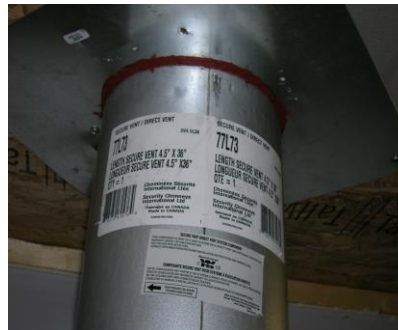
The interior gypsum board, OSB or equivalent is sealed with caulk to the sheet metal flap or fire stop. Seal all joints, seams, and penetrations with caulk or sealant. Seal the sheet metal collar at the flue with fire rated caulk. Maintain all clearances per manufacturer's specifications.
