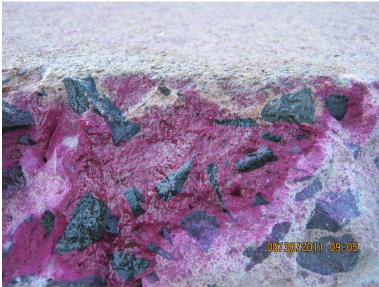
Figure 16. Concrete surface on Level 6 with phenolphthalein applied.
