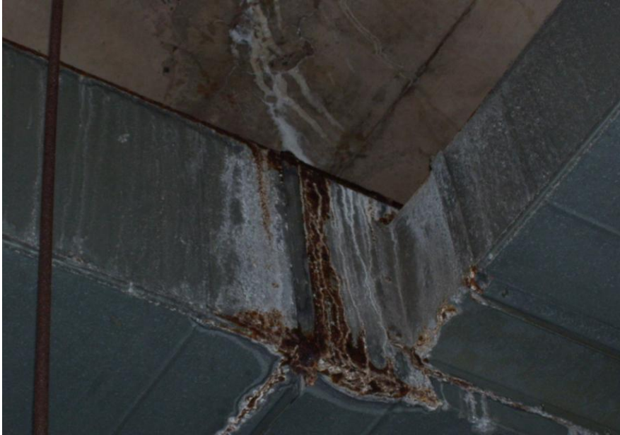
PHOTO 1 Parking Level P3
