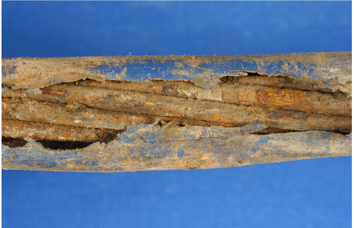
Figure 6. Second location of sheath damage and strand wire corrosion on strand #2.
