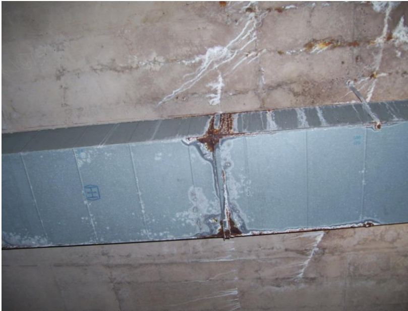
PHOTO 2 Parking Level P3
