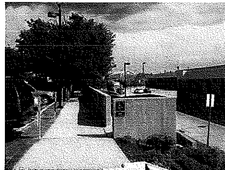
Concrete sidewalk and ramp from upper surface parking lot to GBT Maintenance Facility seen in background (facing east).
