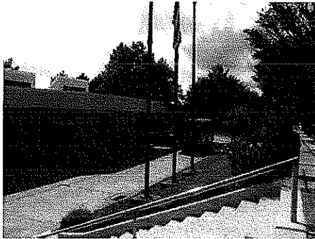
GBT Administration Building and access driveway facing southwest from upper surface parking lot.
