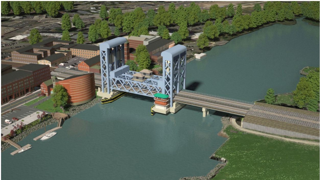
Figure ES-5—Rendering of the Short Span Vertical Lift Bridge in the Closed Position (Option 8A)
