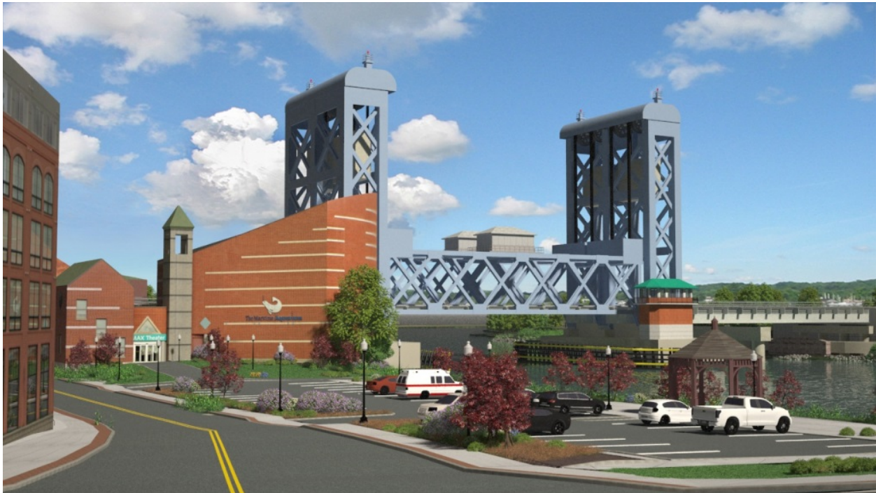
Figure 3-54—Rendering of the Short Span Vertical Lift Bridge (Option 8A) – View from the Southwest
