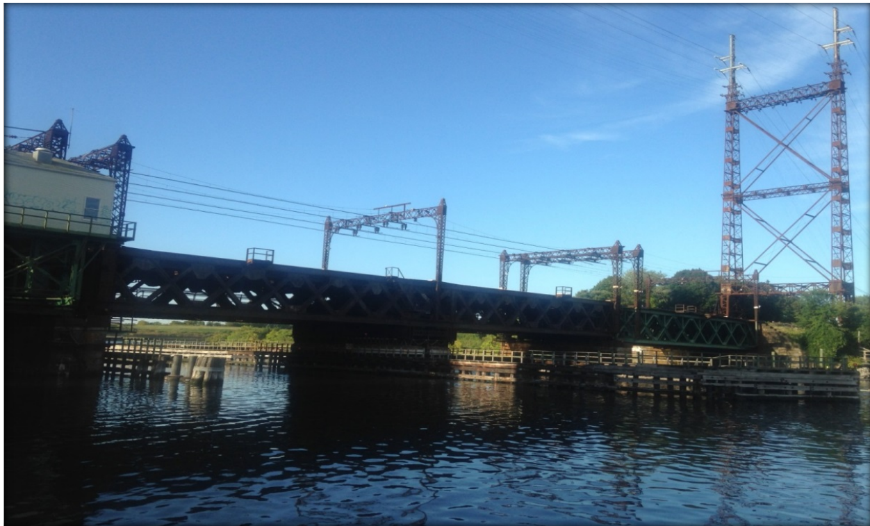
Figure 9-1—View of Walk Bridge, looking northeast
