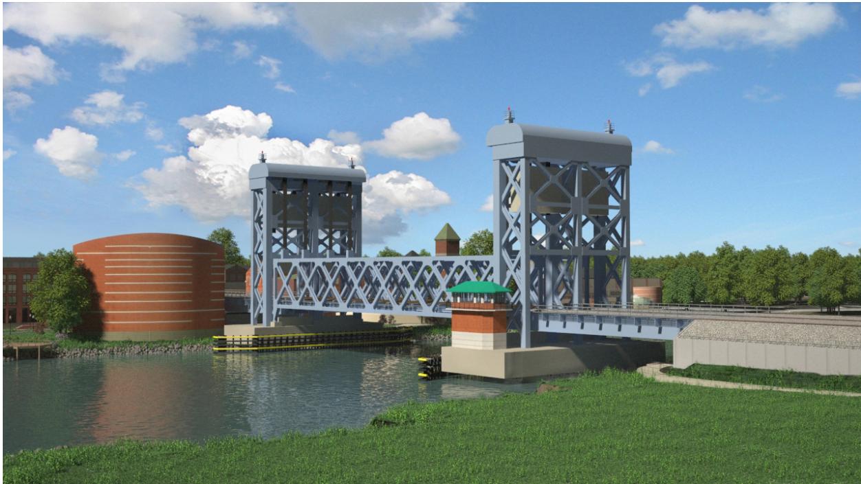
Figure 3-52—Rendering of the Long Span Vertical Lift Bridge (Option 11C) – View from the Southeast
