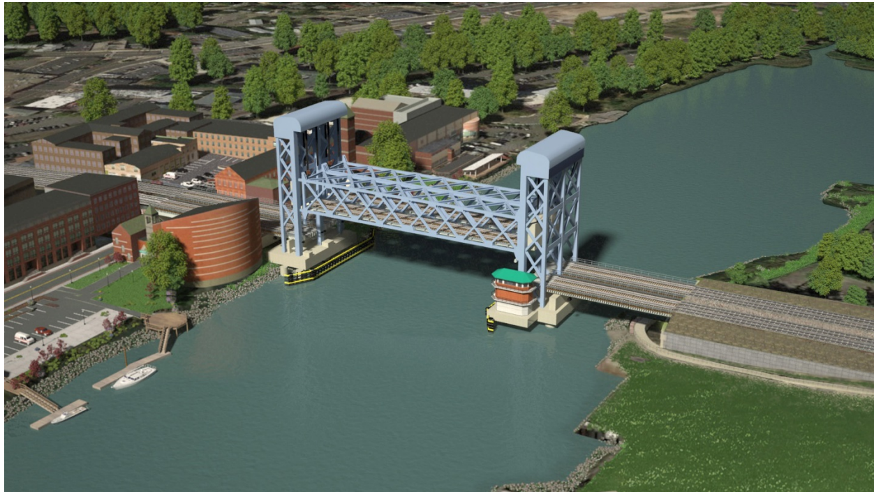
Figure ES-9—Rendering of the Long Span Vertical Lift Bridge in the Open Position (Option 11C)
