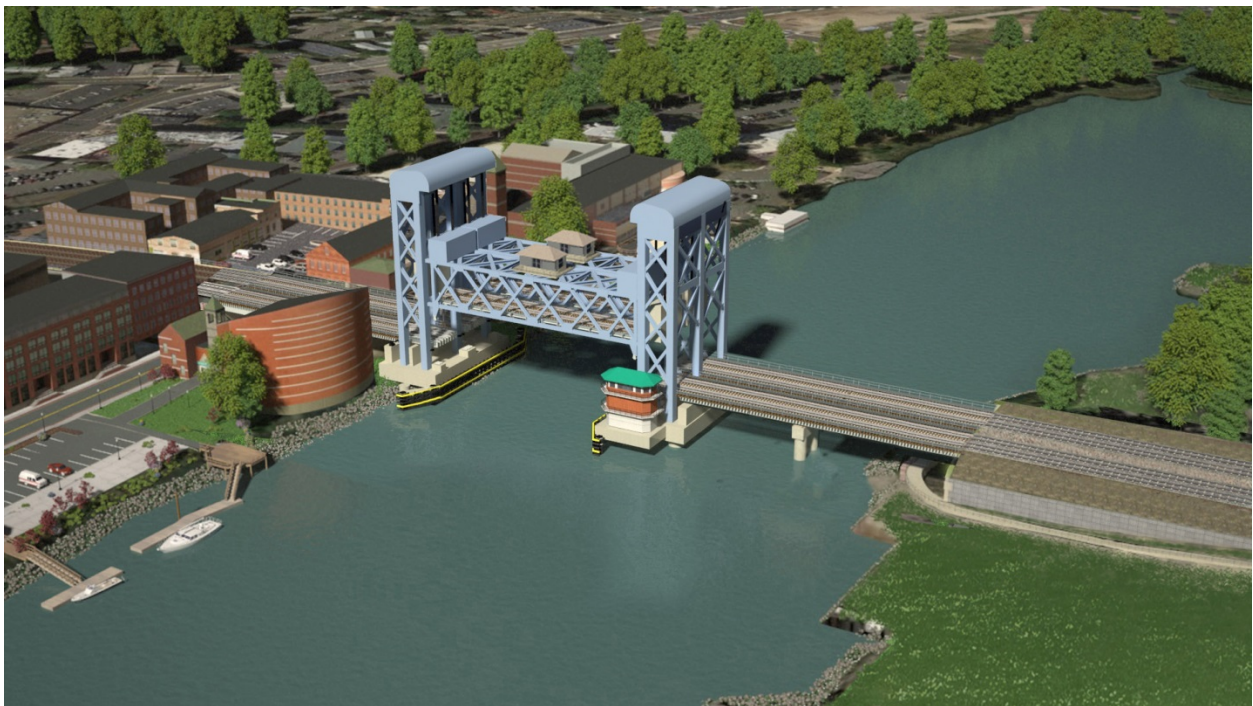
Figure ES-6—Rendering of the Short Span Vertical Lift Bridge in the Open Position (Option 8A)
