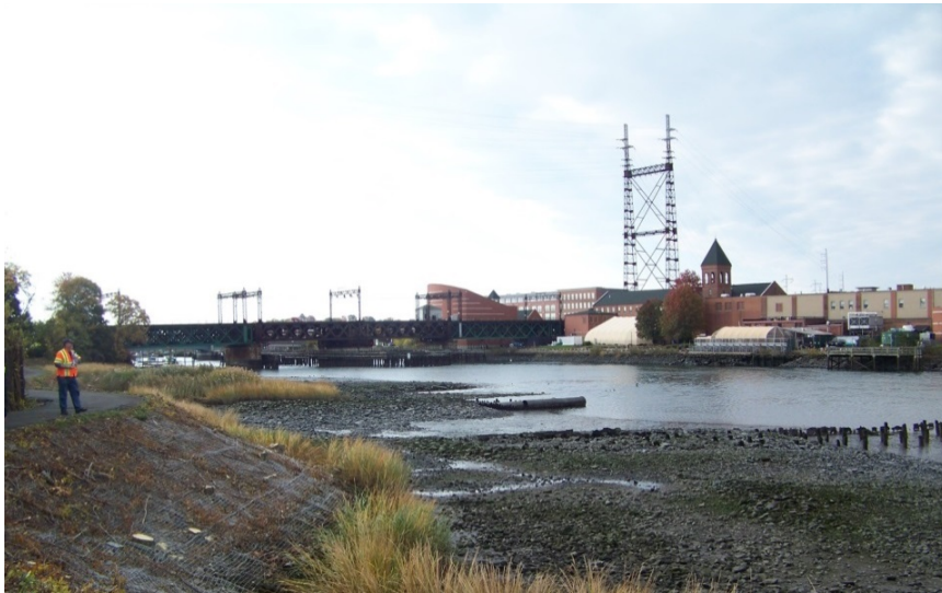
Figure 3-43—View of Walk Bridge, looking southwest from Harbor Loop Trail/Norwalk River Esplanade
