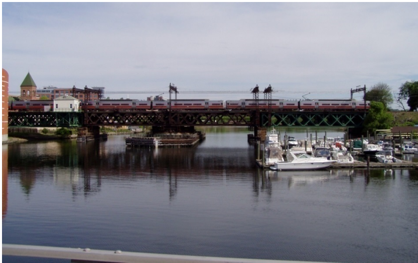
Figure 3-41—View of Walk Bridge, looking north from Stroffolino Bridge
