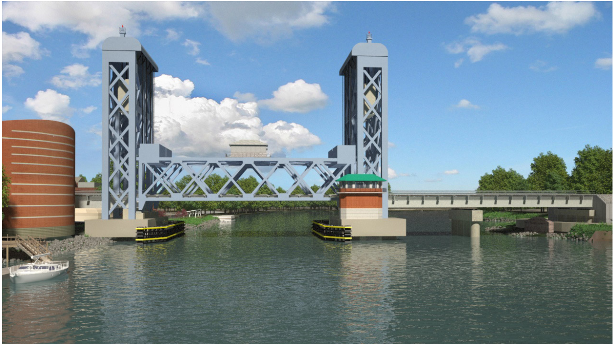
Figure 3-48—Rendering of the Short Span Vertical Lift Bridge (Option 8A) – View from the Water
