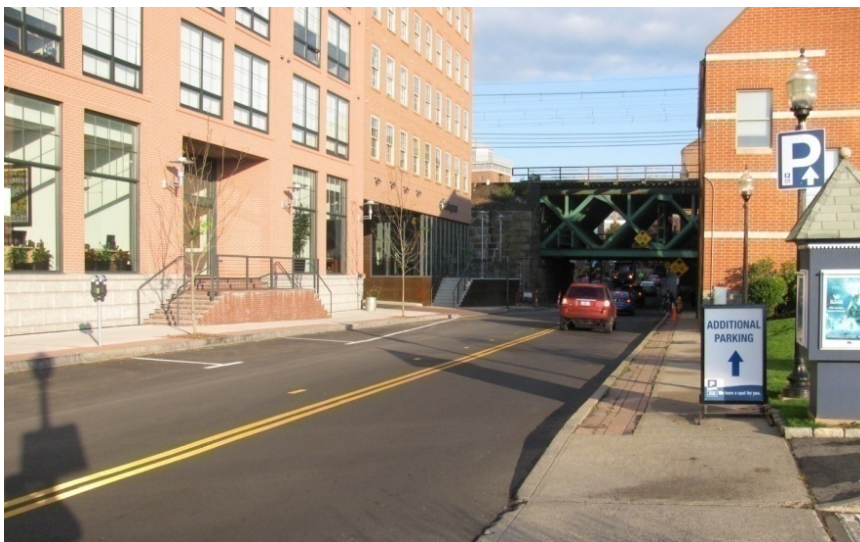
Figure 3-44—View of Walk Bridge west approach, looking north from North Water Street with IMAX Theater on right and Ironworks building on left
