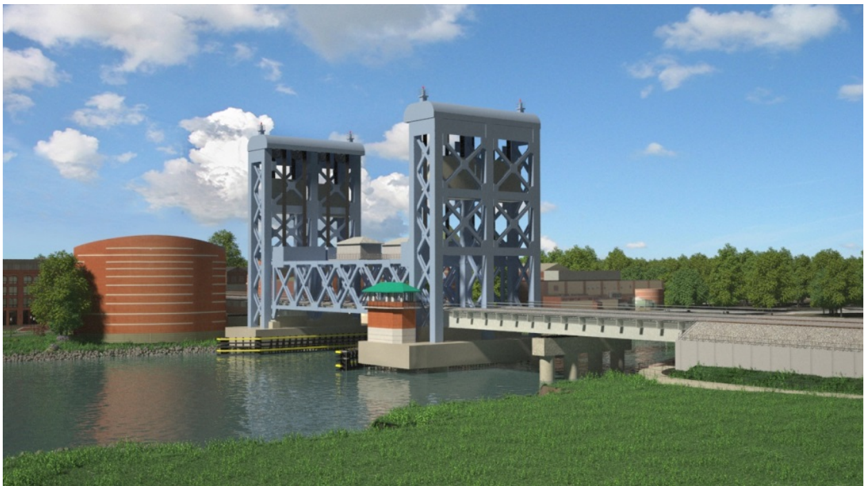
Figure 3-51—Rendering of the Short Span Vertical Lift Bridge (Option 8A) – View from the Southeast
