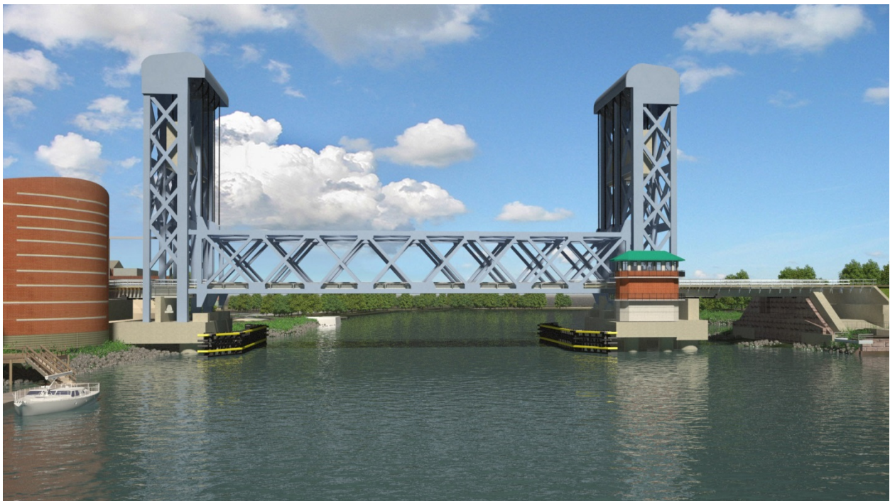
Figure 3-49—Rendering of the Long Span Vertical Lift Bridge (Option 11C) – View from the Water
