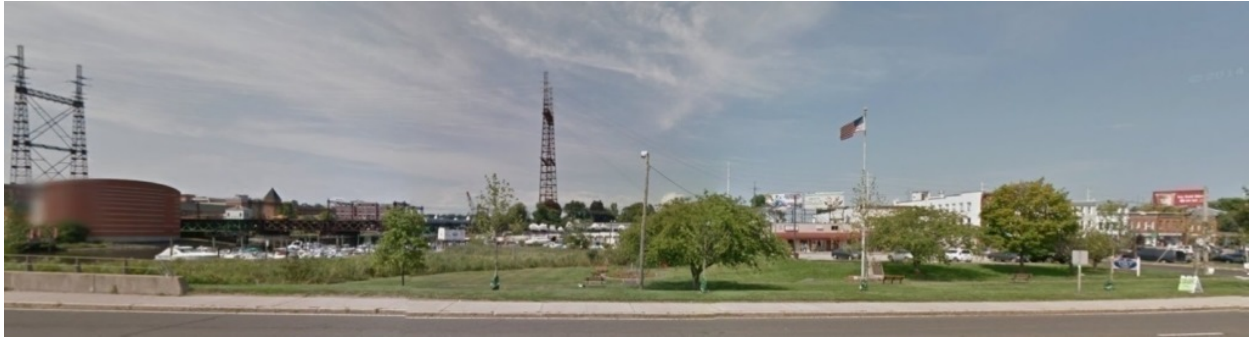
Figure 3-40—View of Walk Bridge, High Towers and Constitution Park, looking northwest from Route 136 (from Google maps)
