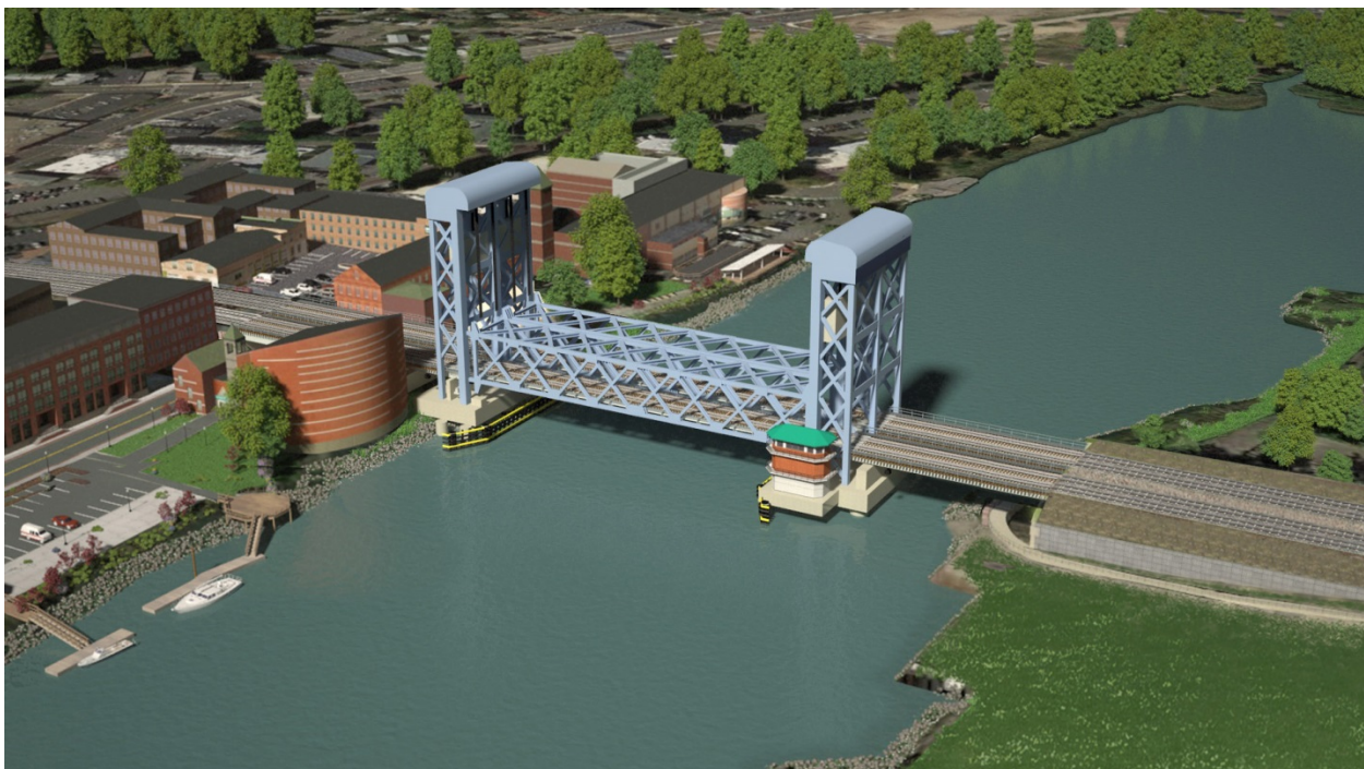
Figure 2-11—Rendering of the Long Span Vertical Lift Bridge in the Closed Position (Option 11C)
