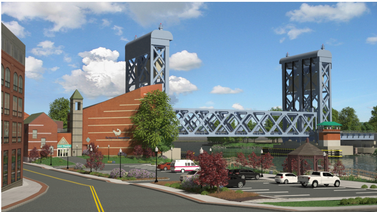
Figure 3-55—Rendering of the Long Span Vertical Lift Bridge (Option 11C) – View from the Southwest
