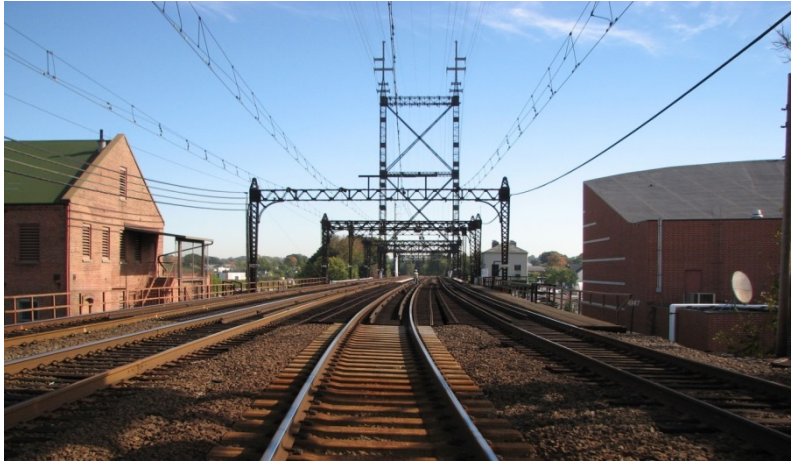
Figure 3-34—View of Walk Bridge, looking east from railroad with Maritime Aquarium on left and IMAX Theater on right
