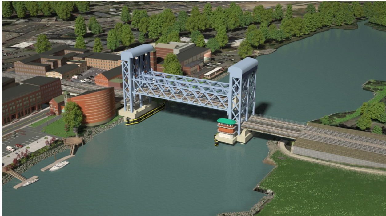
Figure 2-12—Rendering of the Long Span Vertical Lift Bridge in the Open Position (Option 11C)
