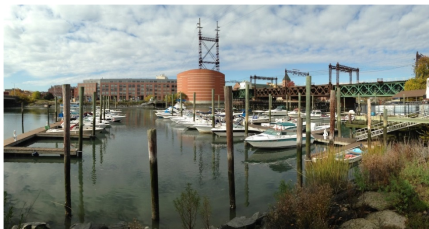
Figure 3-38—View of Walk Bridge and West High Tower, looking northwest from private marina in East Norwalk
