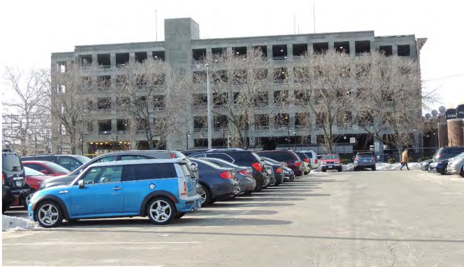
Exhibit 3.9-2: View South Across the Project Site to the Union Station Parking Garage
