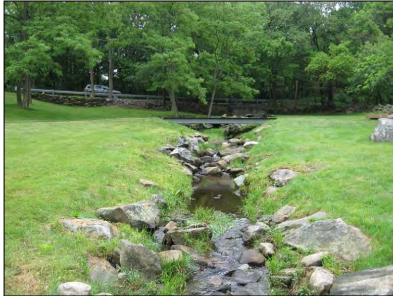
Stream segment GB-05B showing limited vegetative buffer and a small footbridge crossing the stream.
