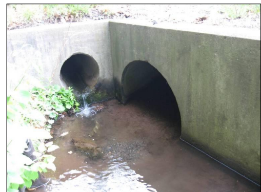
Stream crossing (SC-01) below I-84 and outfall (OT-03) along reach GBST-02.
