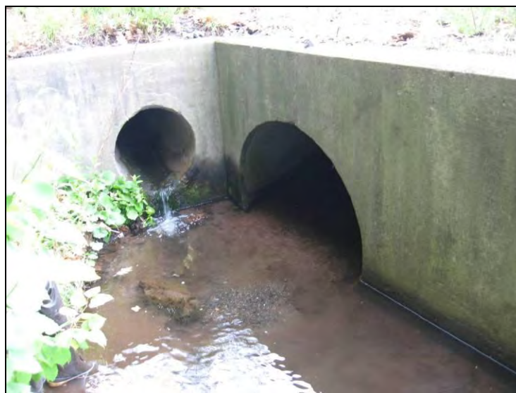
Stream crossing (SC-01) below I-84 and outfall (OT-03) along reach GBST-02.
