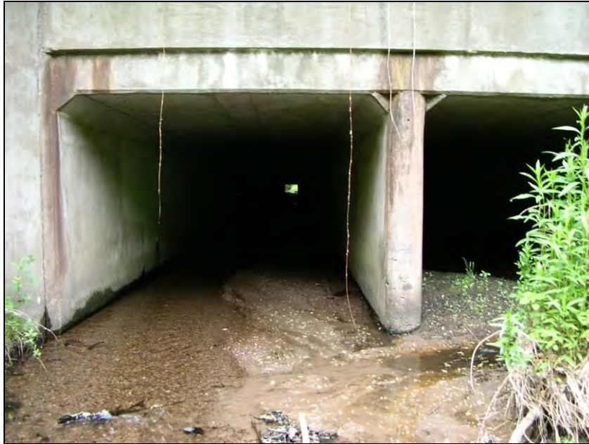
Twin box culvert along reach VWR-05 underneath the onramp for I-84.
