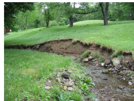
Streambank erosion along Gages Brook.
