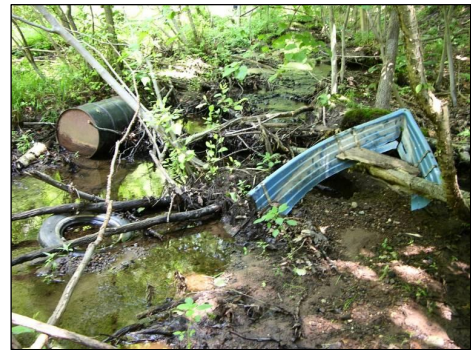
Trash and debris along Reach CB-02.
