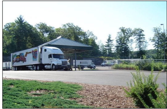
The Dari Farms Ice Cream Distribution Facility has a covered fueling station and landscaped grounds (shown in the foreground).
