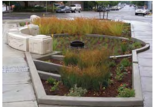
Figure 6-2. Rain garden in an urbanized area. Source: Portland River Renaissance Initiative
