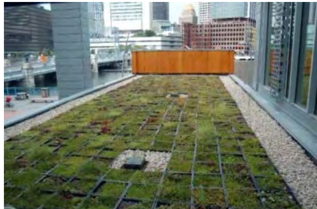
Figure 6-8. Green Roof at the Children's Museum in Boston, Massachusetts. Source: Photo provided by laurenmetter.com
