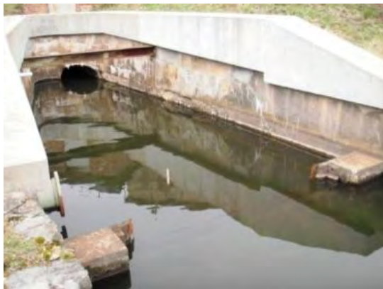
Figure 6-11. North Stamford Dam low flow outlet
