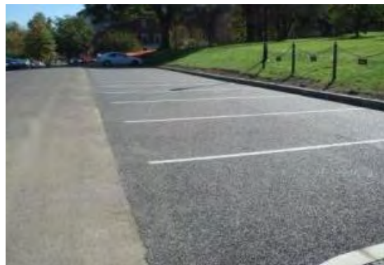
Figure 6-6. Porous pavement parking lot constructed as part of the CDM Smith Hartford Green Capitals Project
