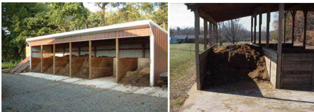
Figure 3-2. Examples of covered manure storage facilities (left - Rutgers Equine Science Center, Rutgers University; right - Michigan State University Extension)
