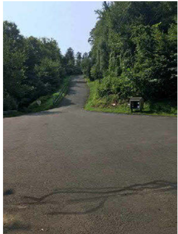
Figure 8: View of Pascoe Drive from the cul-de-sac looking up the hill. Potential opportunity for stormwater BMPs in the cul-de-sac or beneath it.
