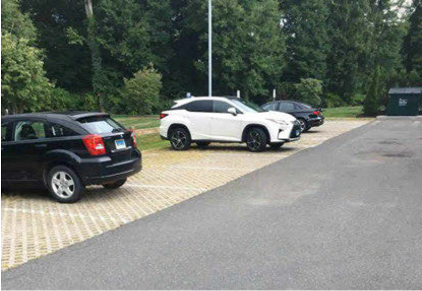
Figure 9: Example of pervious parking surface behind commercial plaza at 7 Garage Road, Southbury.
