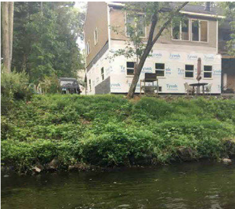
Figure 6: House with limited buffer to Pomperaug River encountered during stream walk.
