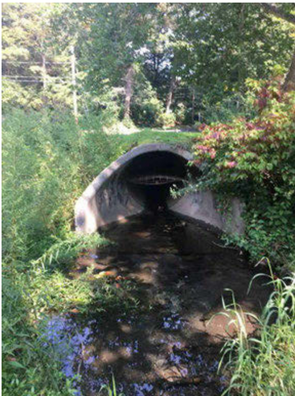
Figure 3: Stormwater outfall at Cedarland Park off of River Trail Road.
