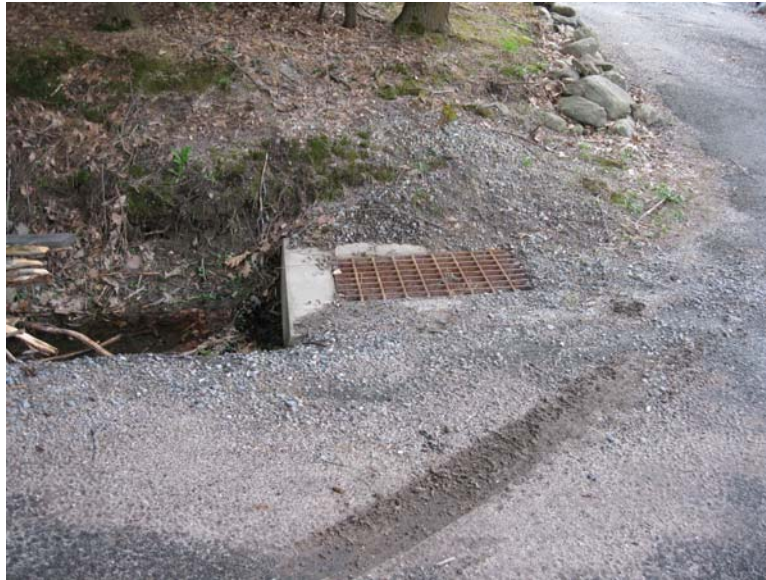
Install Large Particle Separator
