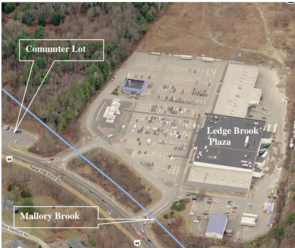
Figure 4 – Ledge Brook Plaza and State Commuter Parking Lot
