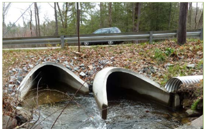
Figure 2 West Hill Road Structured Stream Crossing
