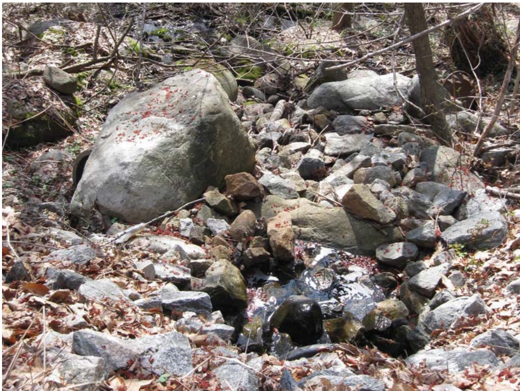
Outfall below Ricki Road
