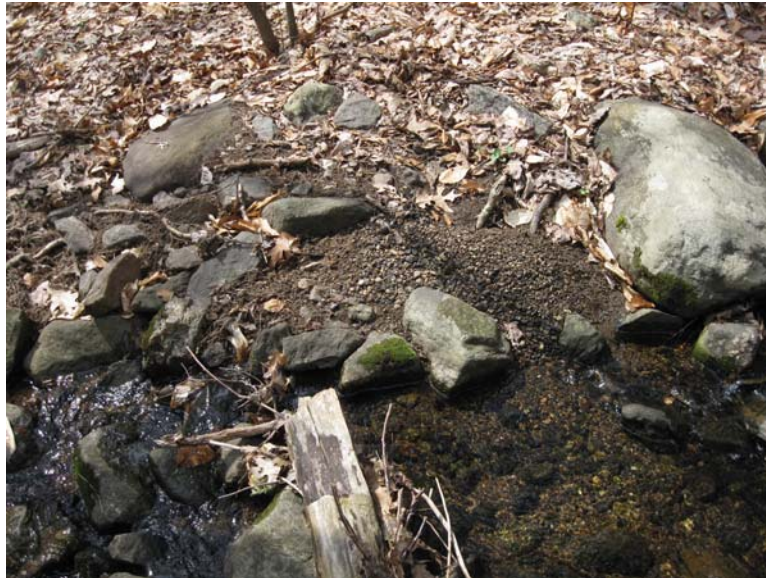
Evidence of Active Erosion that Progressively Moves Toward Pond
