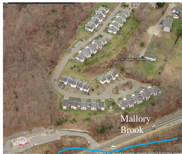
Fig- 3 Green Ridge Condominium and Former KFC Restaurant
