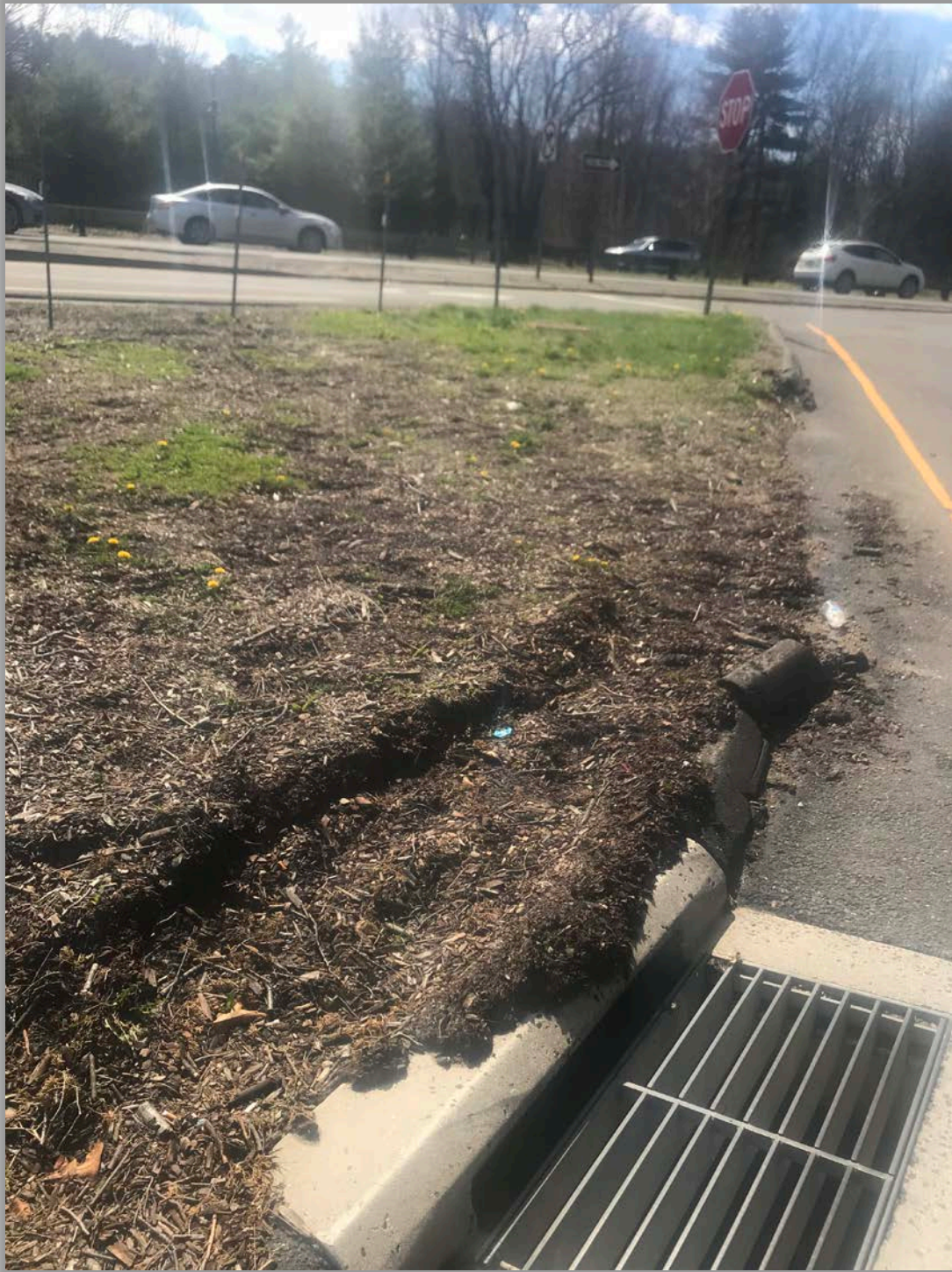
Figure 5.31: Candidate site for tree filter install to improve interception of stormflow, reduce delivery of solids such as mulch to catch basins, and remove bacteria
