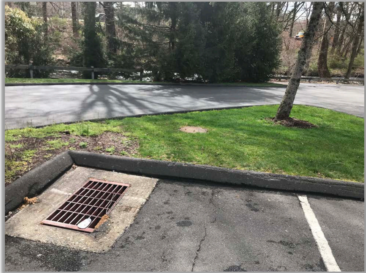
Figure 5.29: Target area for tree well unit; existing catch basin offers no stormwater treatment
