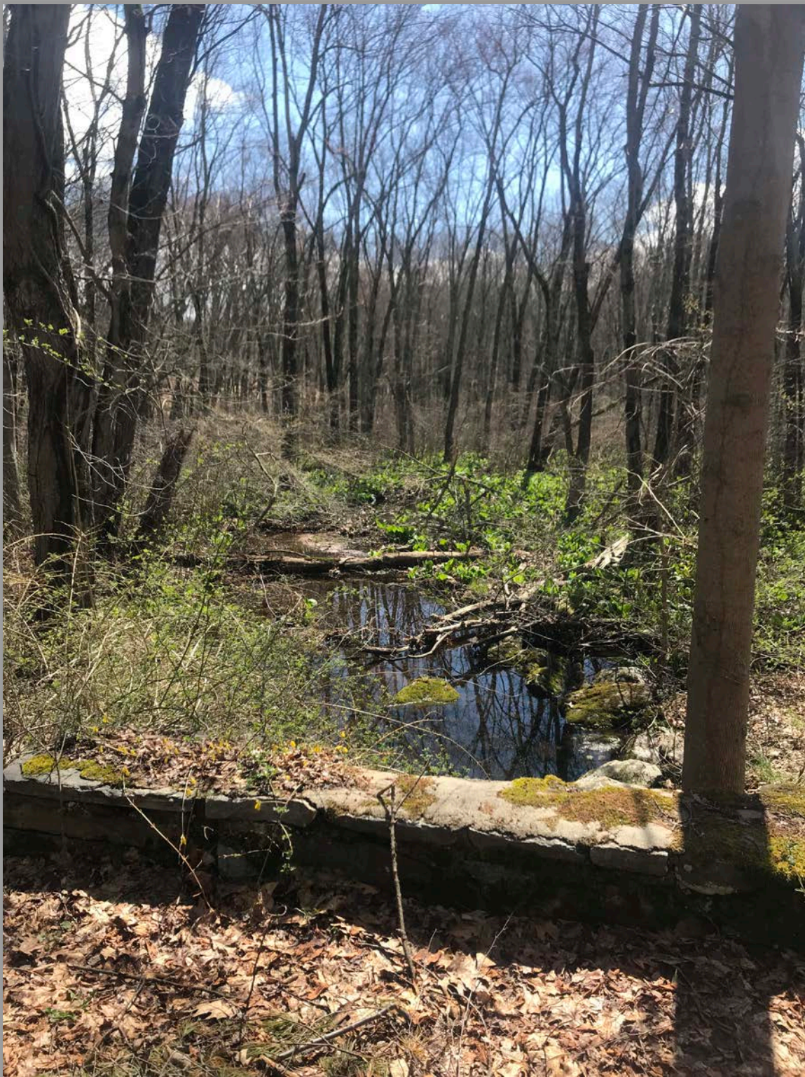
Figure 5.48: Catch basin discharges to Morehouse Brook at the road culvert creating bank instability and downstream sedimentation
