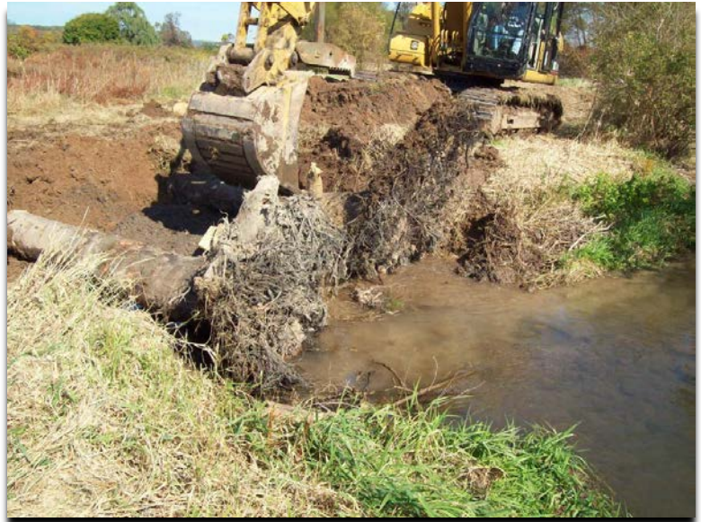
Figure 5.17: Rootwad Placement. Source: Princeton Hydro
