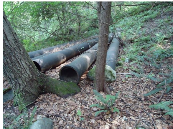
Photo 87: abandoned iron pipes associated with the water line right-of-way
