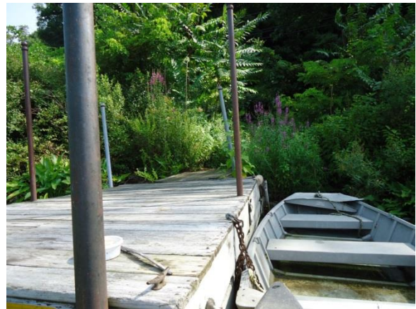
Photo 317: Dock along segment HP-06/07
