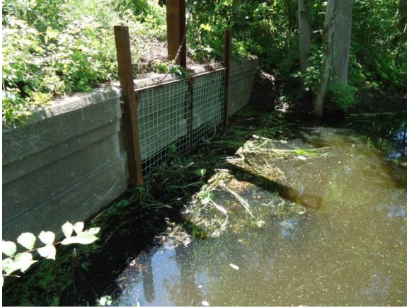
Photo 56: Box culvert stream crossing for South Kent Road and Womenshenuk Brook
