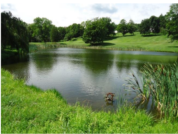
Photo 17: Outlet structure in School Pond
