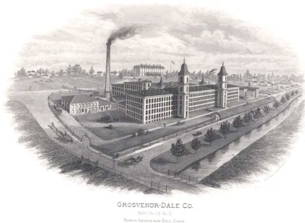
Figure 3-5. The Grosvenor-Dale Mill in the village of North Grosvenordale circa 1872-1896. The French River is visible on the right side of the image.
