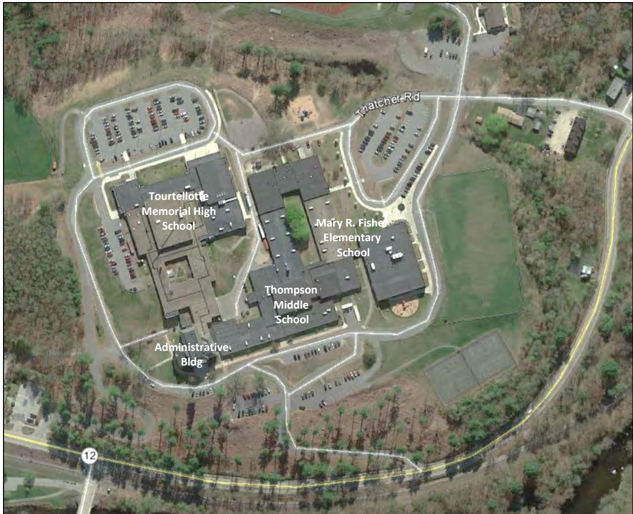
Figure 8-29. The Thompson public school complex on Riverside Drive (RT 12) and Thatcher Road in North Grosvenordale (Google Earth imagery dated 5/6/15).
