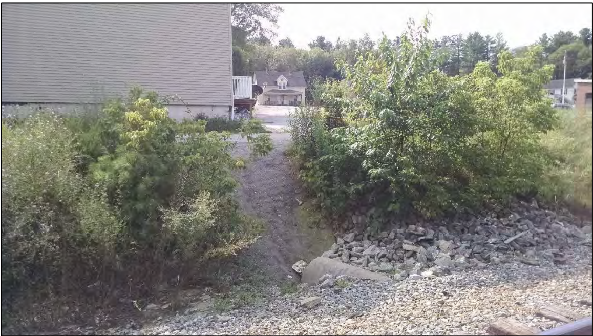
Figure 8-21. One of three leak-offs from Market Street onto the P&WRR ROW.
