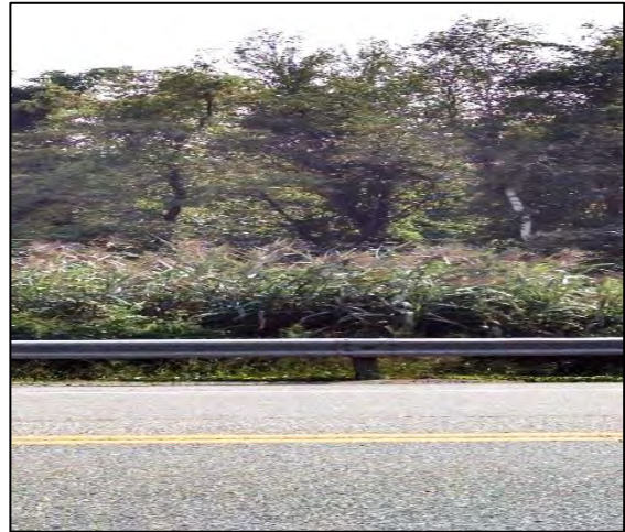
Phragmites growing at a stormwater outfall along Route 12 near the French River.
