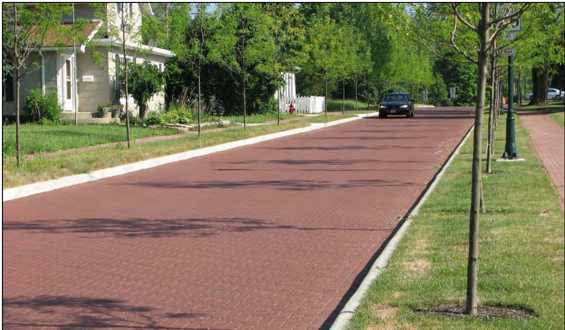
Figure 8-12. A residential pervious paver road (Image from Pine Hall Brick Company, Inc. www.pinehallbrick.com ).
