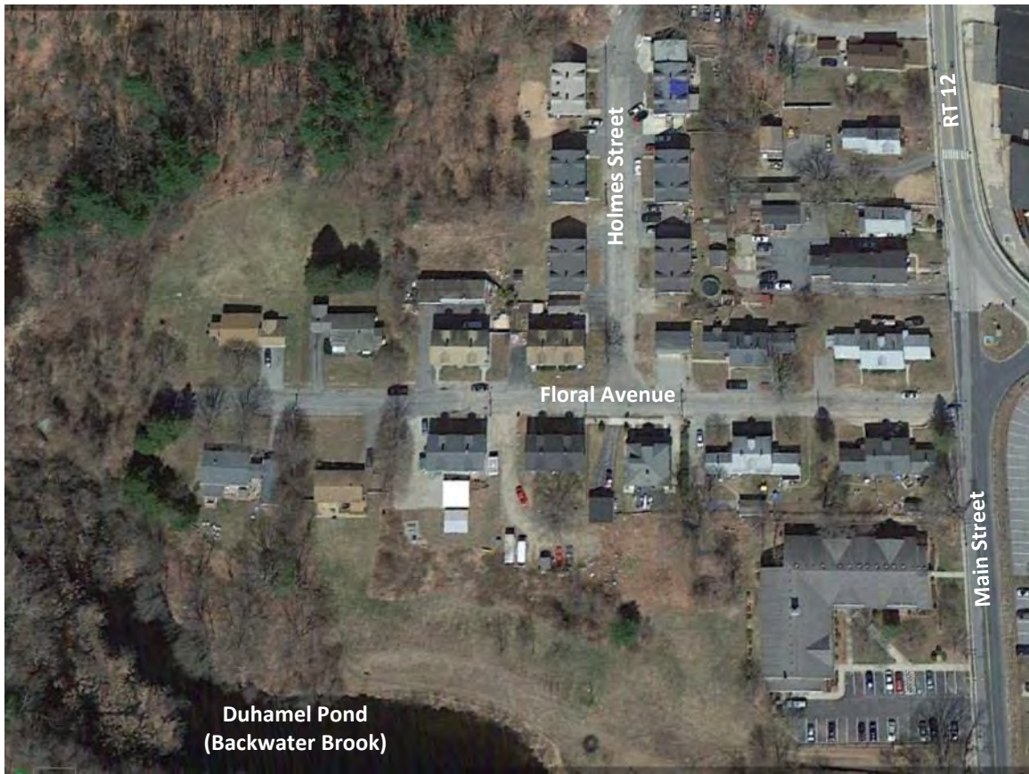
Figure 8-10. Swede Village, located on Holmes Street and Floral Avenue, is typical of late 18 th century former mill housing found throughout the mill village of North Grosvenordale (Google Earth imagery dated 4/7/13).
