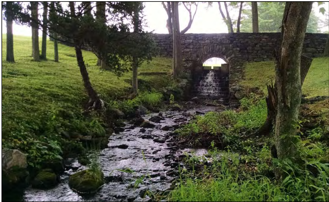
Figure 3-24. Dam on Quinatissett Brook at the outlet of Reams Pond.
