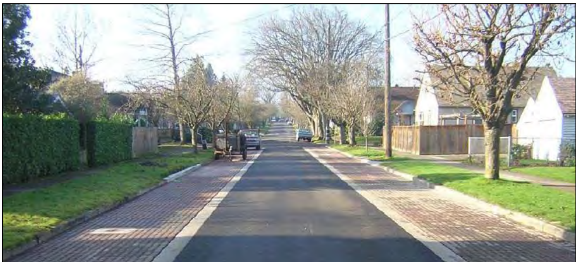
Figure 8-9. Example of a roadway with pervious paver shoulders (from LID Appendix to CT Stormwater Quality Manual, 2011).
