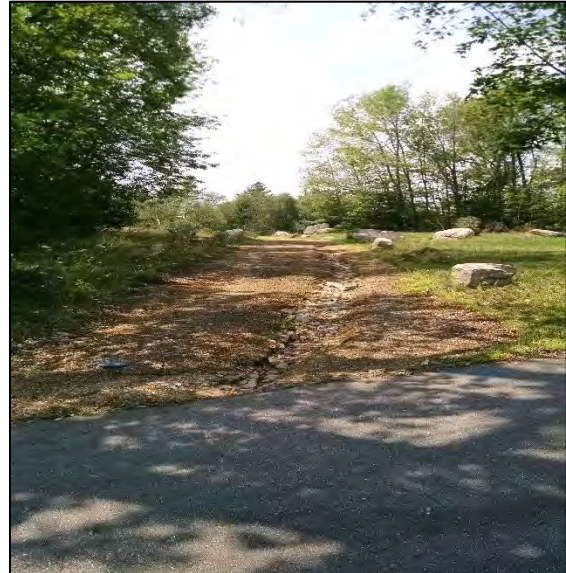
Uncontrolled stormwater runoff from a commercial property in North Grosvenordale has resulted in the development of a deep gully and deposition of the eroded sediment in the street down-gradient of this dirt driveway.
