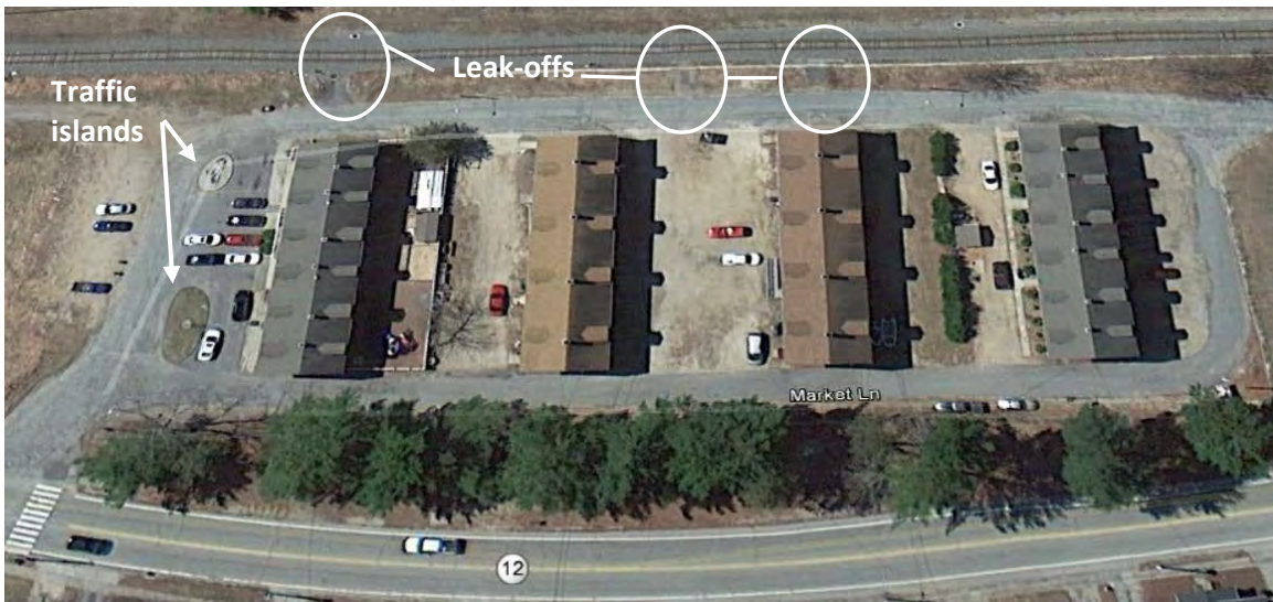
Figure 8-19. Aerial image of Greek Village, located off RT 12 in North Grosvenordale (Google Earth imagery dated 4/7/13). The leak-offs from Market Street onto the P&WRR ROW are delineated by the white circles.
