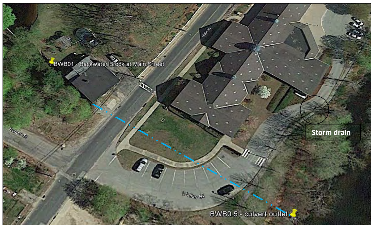
Figure 31. Culverted segment of Backwater Brook (dashed line). Approximately 250 feet of the stream is culverted under Main Street and the Thompson Public Library property.
