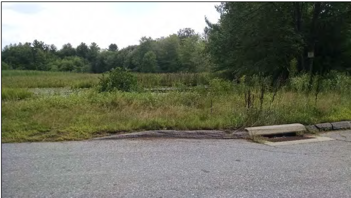
Figure 5-6. Stormwater from Wilsonville Road discharges directly to this small pond without any water quality treatment.
