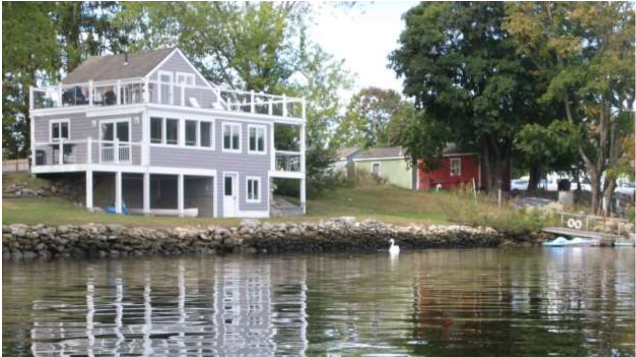
Figure 8. Lack of riparian buffer offers little opportunity for stormwater to be slowed down and infiltrated into the ground. Additionally, the removal of riparian vegetation often results in the need to install hard structures like this stonewall to prevent shoreline erosion.
