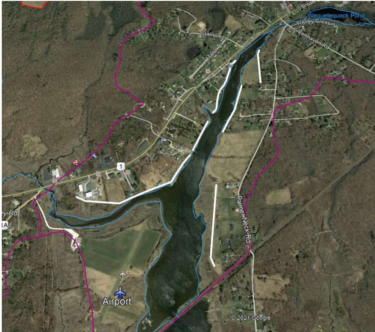
Figure 7-2. Recommended BMPs along the Wequetequock Cove shoreline. The proposed locations of permeable reactive barriers are depicted by the white lines (Google Earth, imagery date 4/22/2018).
