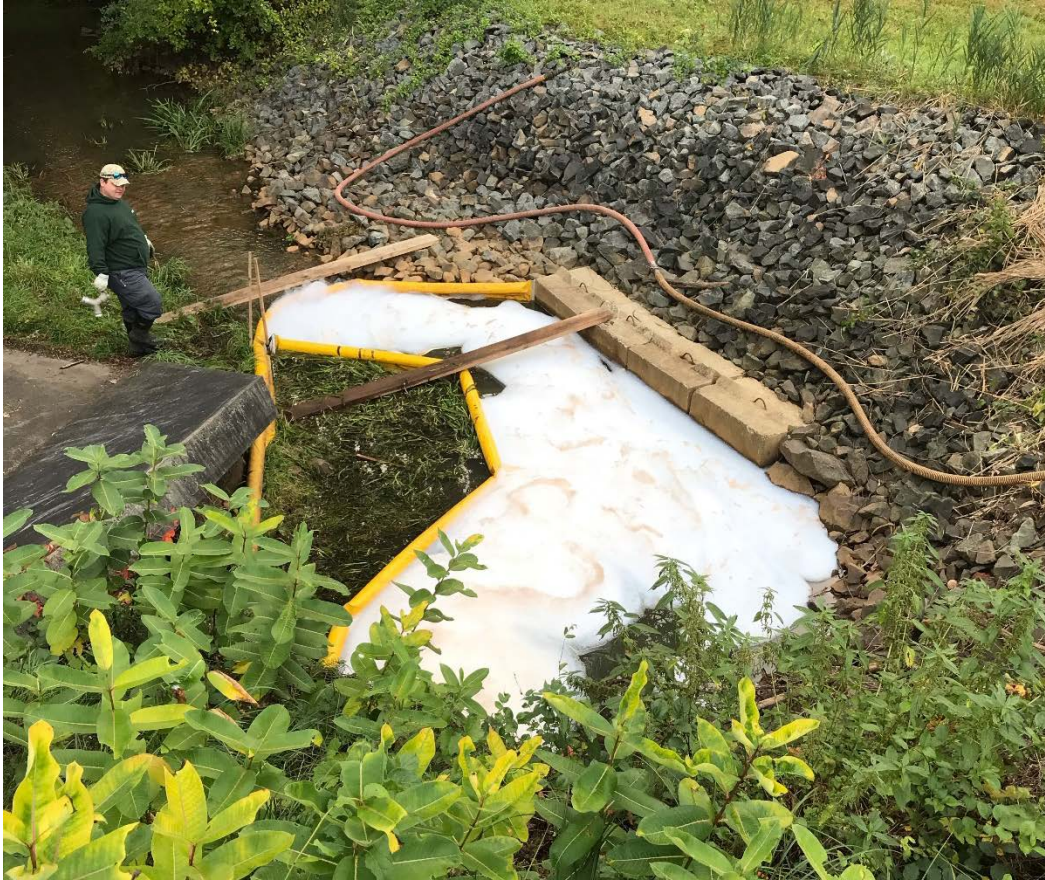
Downstream of Hamilton/Watts Pond Dam
