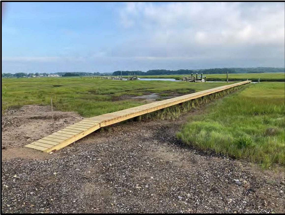
View of project site looking northwest.
