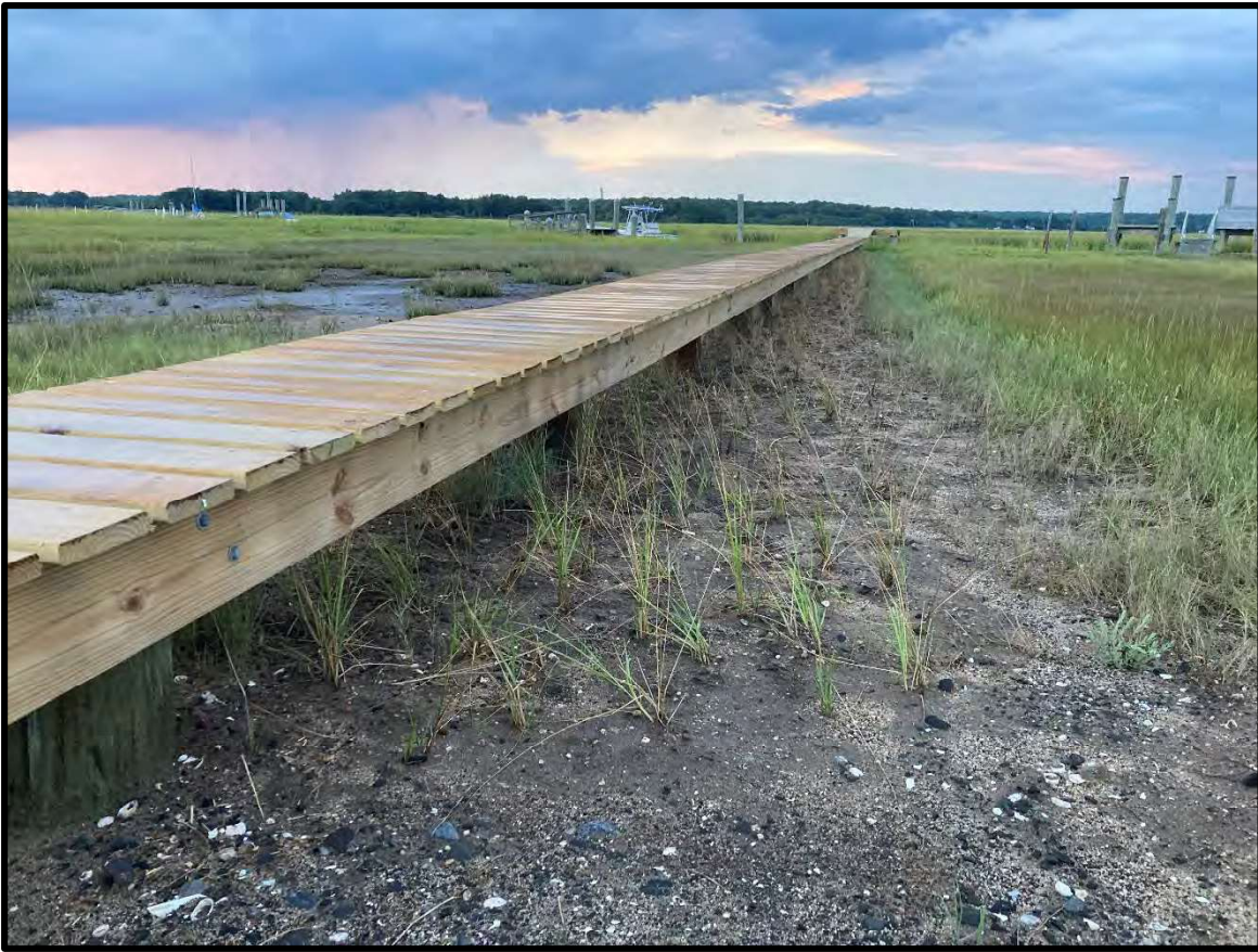
View of project site looking northwest.
