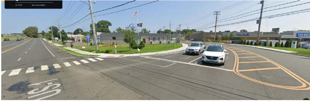
After - Reconstruction of Interchange 33 on Interstate 95 (Courtesy: Google Maps).
