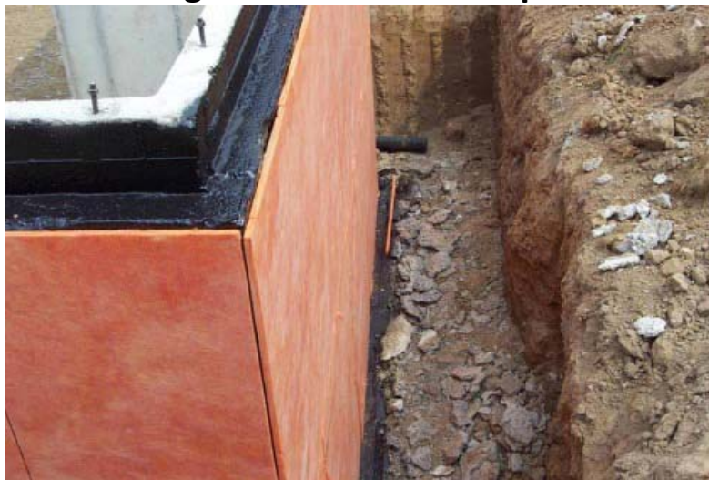
Below-grade wall insulation R-value. Installed per manufacturer's instructions.
