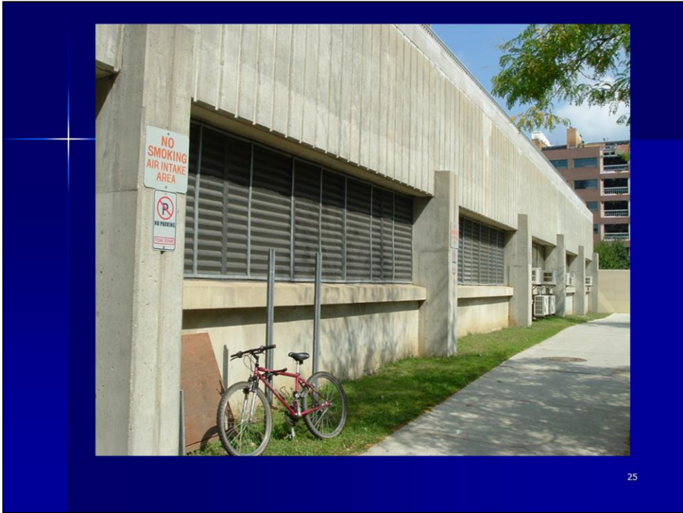
Air intake for ventilation system at grade
