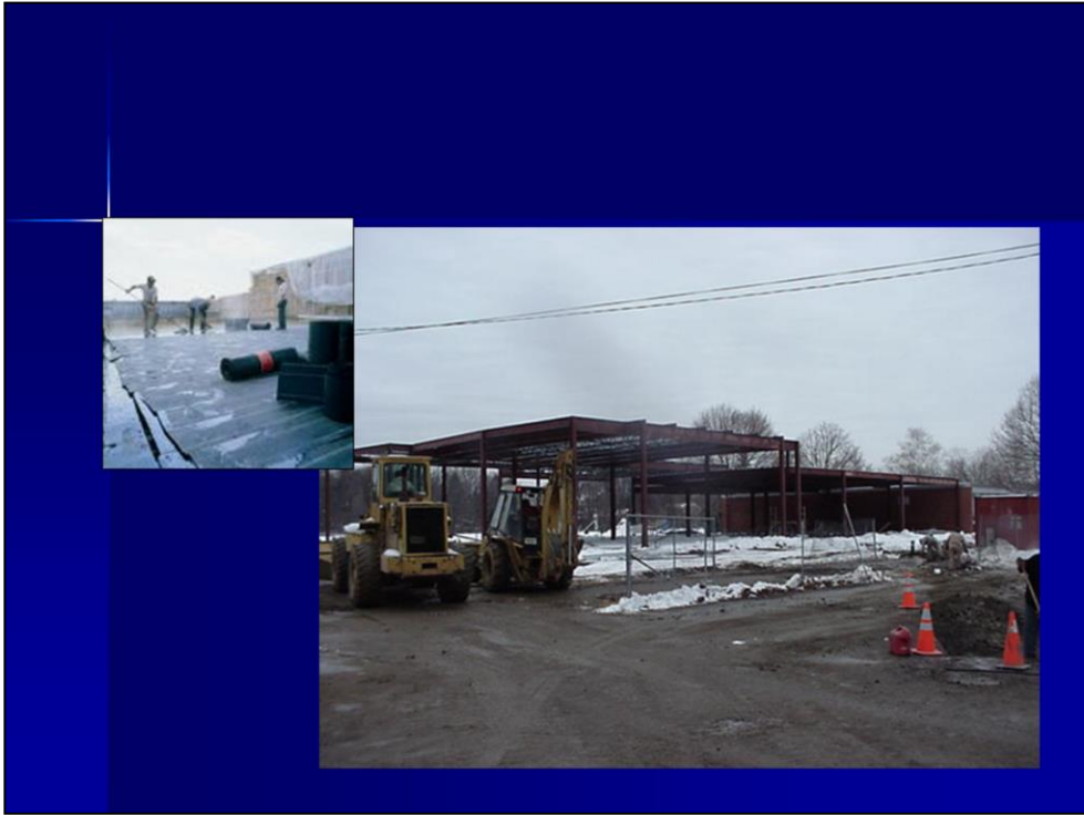
Occupied buildings under construction
