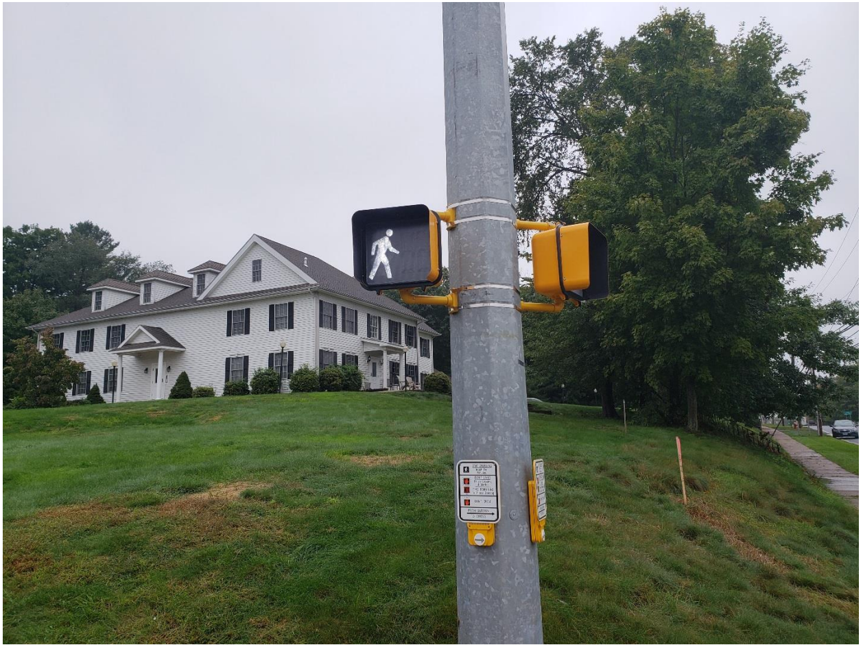
Figure 10: Walk symbol indication, APS pushbutton, and pedestrian sign provided with exclusive and concurrent pedestrian phasing
