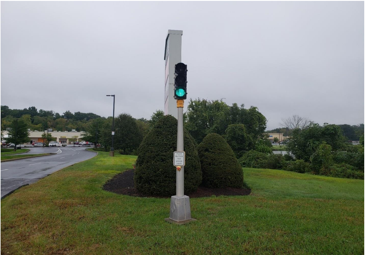
Figure 9: Side street green indication
