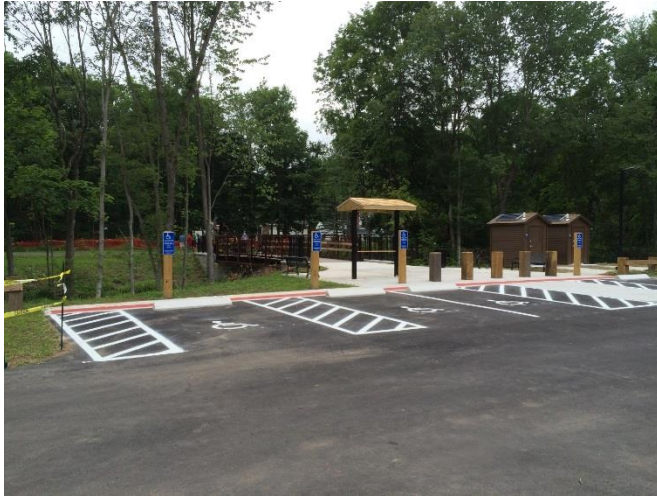
Figure 15: Recently constructed trail head parking located along the Farmington Canal Heritage Trail at Jarvis Street in Cheshire. Typical accessible elements include parking spaces, paths, ramps with tactile warnings, signage, and markings. Photo July 2016
