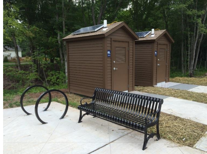
Figure 16: Recently constructed ADA accessible restroom facilities along the Farmington Canal Heritage Trail at Jarvis Street in Cheshire. Photo July 2016
