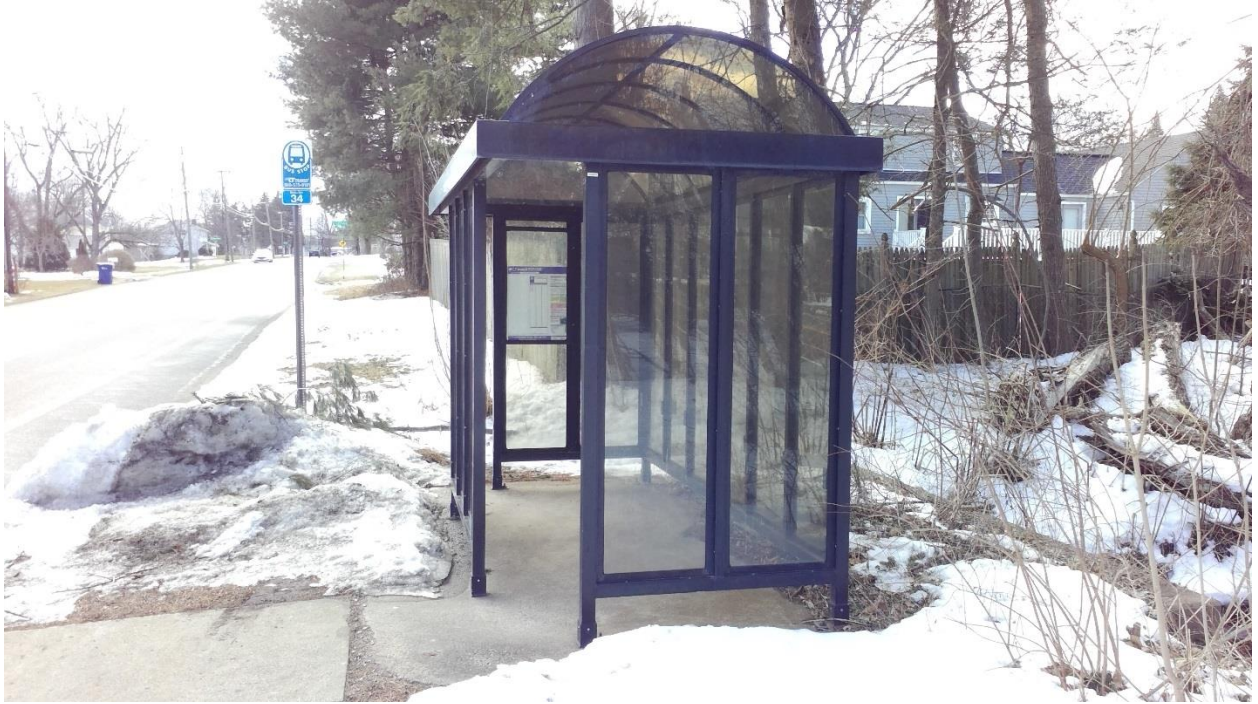
Figure 13: Bus Shelter on Eastview Drive in Windsor (2019)
