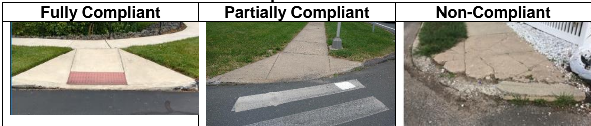
Figure 7: Curb Ramp Condition Definition
