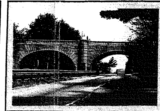
Bridge Framing Views - James Farm Road Bridge (NB)
