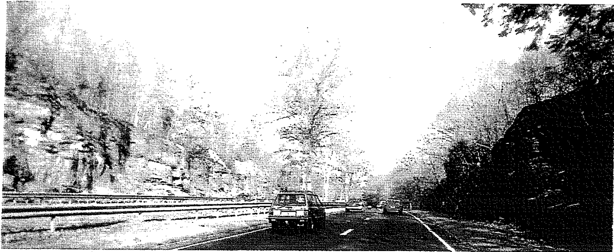
STATION 145+000 LOOKING EAST
