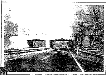
Bridge abutment revealed nicely through trees
